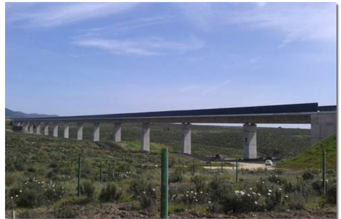
AVE CAÑAVERAL RAILWAY BRIDGE. Spain.
