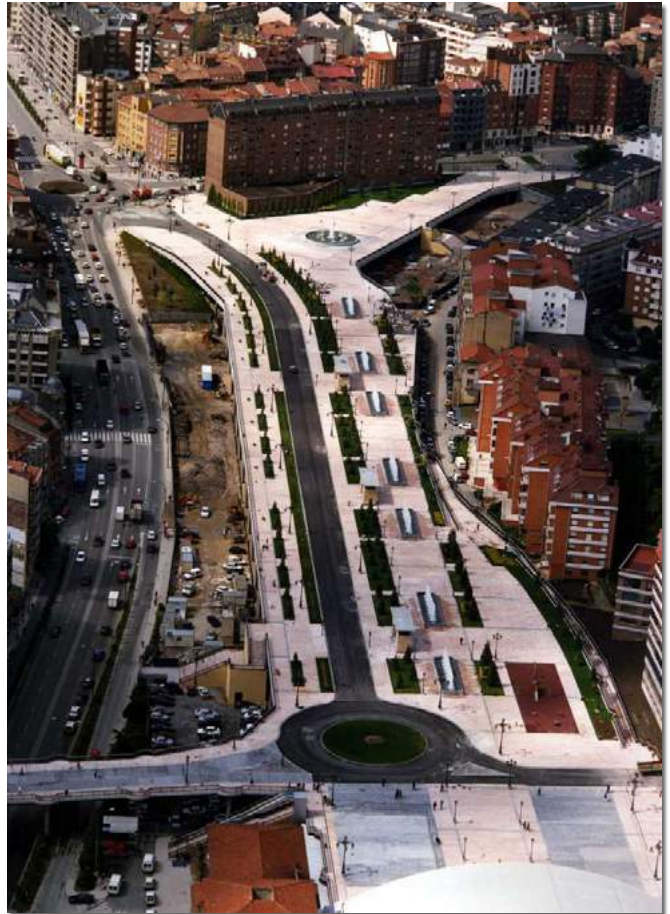
RAILWAY STATION IN OVIEDO. Spain.
