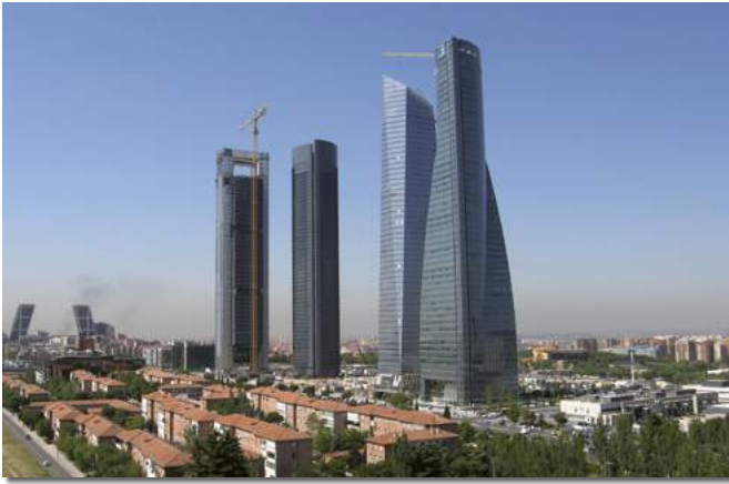
MADRID TOWERS. Spain.
