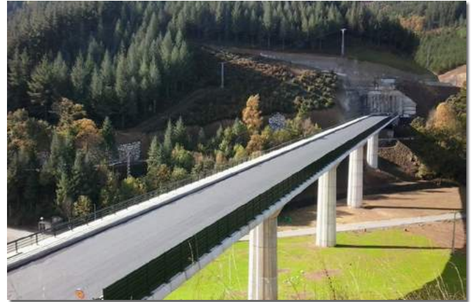
AVE BEASAIN RAILWAY BRIDGE. Spain.
