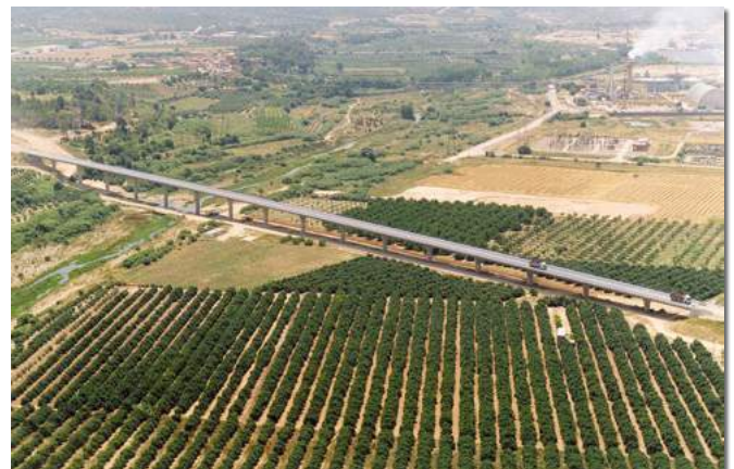
AVE TARRAGONA RAILWAY BRIDGE. Spain.
