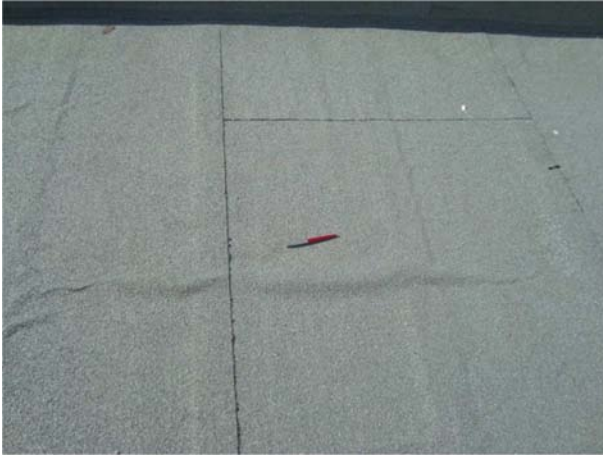
Wrinkles perpendicular to the longitudinal direction of the roll.
