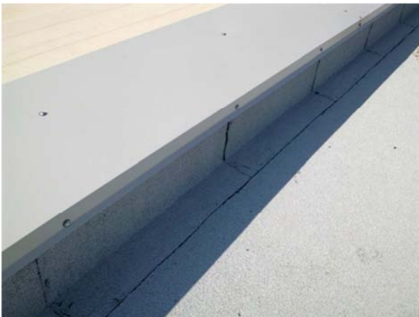
Metallic coping at a low upstand of a roof.
