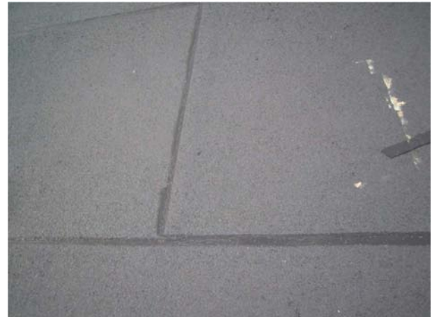
Longitudinal and transversal overlap retraction.
