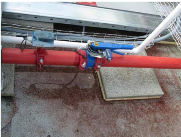
Duct support element retaining water drainage.
