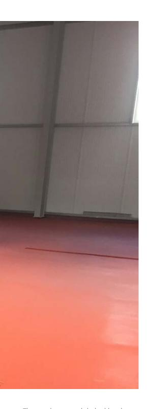
The result is a solid, highly elastic, solvent- and plasticiser-free membrane with 100% solids content, curing in seconds, continuous, without the need for joints or overlaps, which fully adheres to a wide variety of substrates, both horizontal and vertical, and which adapts to different geometries, however complicated they may be.
