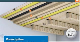
Refurb of residential buildings, public and commercial ground-floor buildings with exposed wooden structures. The membrane between panels improves the insulation for low frequencies by displacing resonant frequencies. It does not require a protective layer against humidity. Thin solution.
